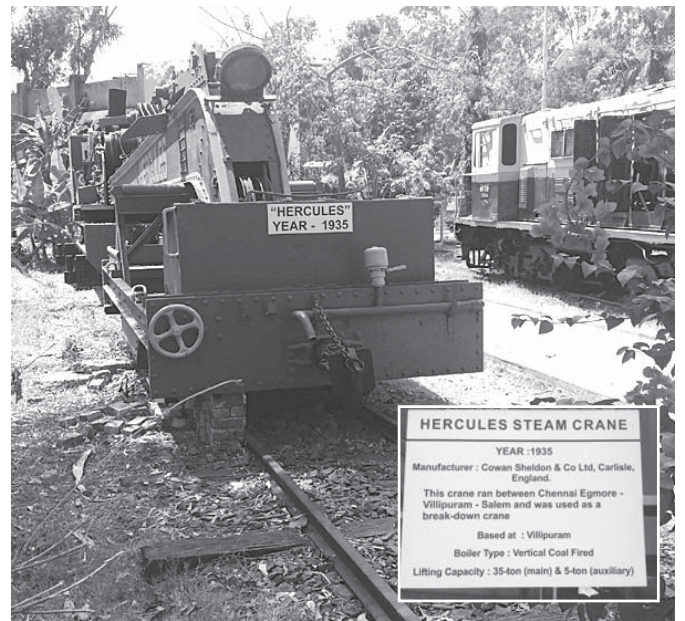
The 1935 built Hercules steam crane for rescue operations, seen on location. Inset: Details of Hercules crane.
