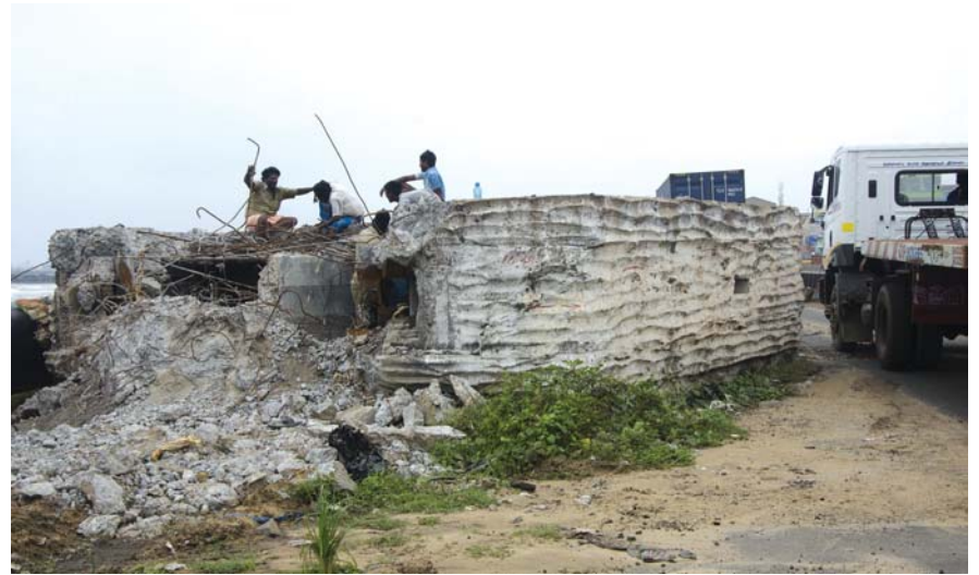
Work on demolishing the World War II air raid shelter in Royapuram. (Photograph: Shantanu Krishnan.)
