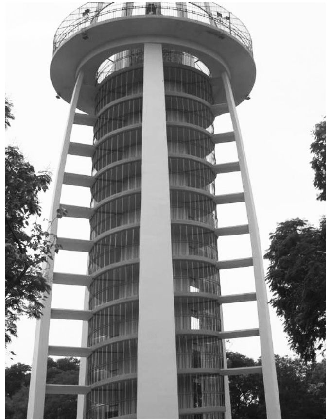
Anna Nagar Tower. Picture courtesy: The Hindu.
